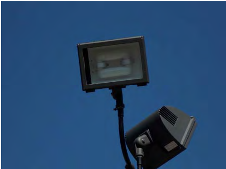
This is an induction lamp with a rectangular profile.
