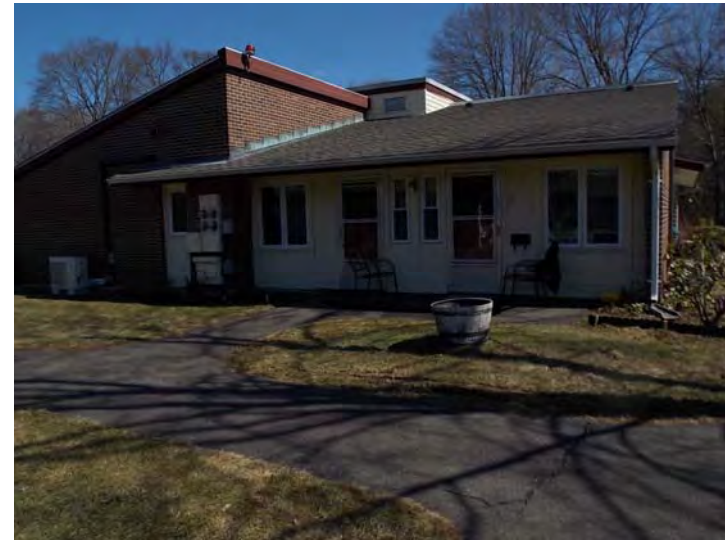
The residential buildings have wood (on right) and brick siding.
