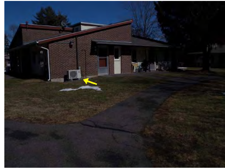
Each apartment has its own heat pump (arrow).
