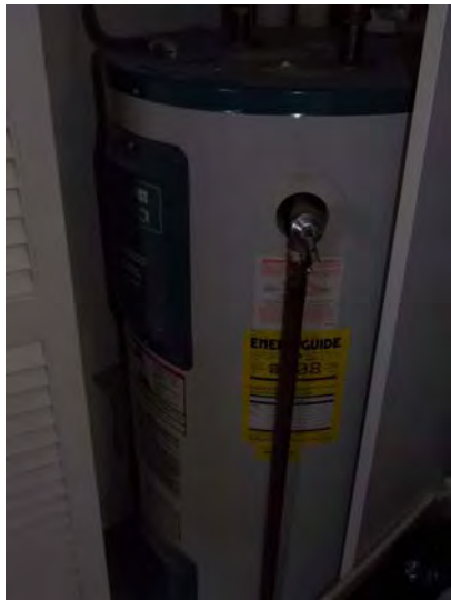
Each apartment has an electric-heated DHW tank.
