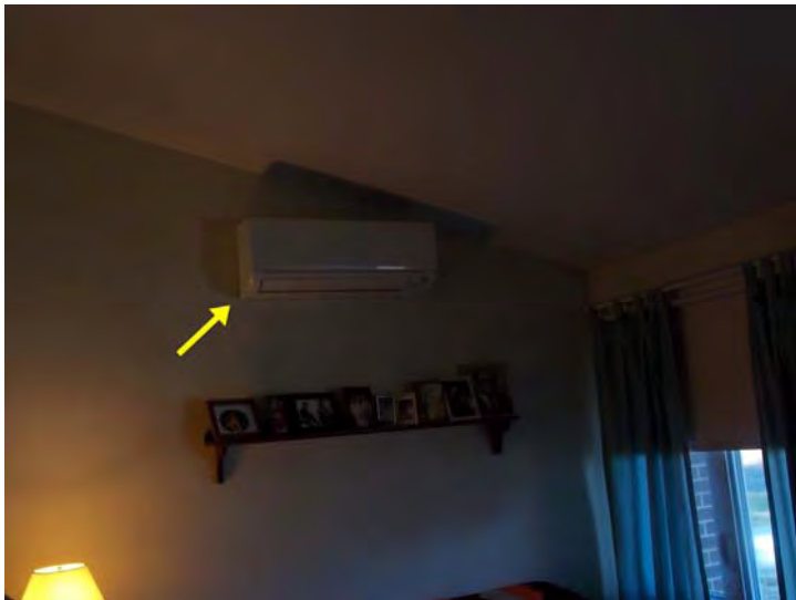
One of the wall-mounted heat pump terminal units.
