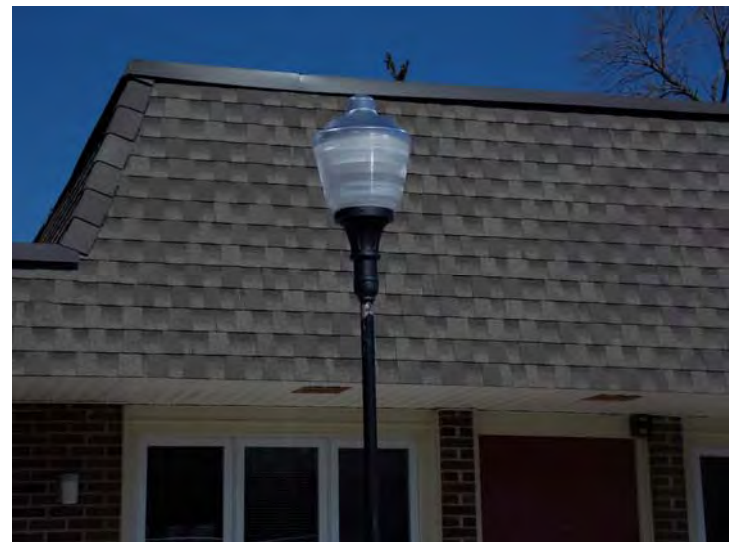
The pole-mounted lighting has been upgraded with induction lamp fixtures, which use 65 watts of power.
