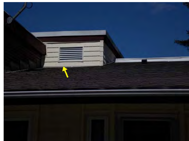
The small attic area on the residential buildings is clad in vinyl siding.
