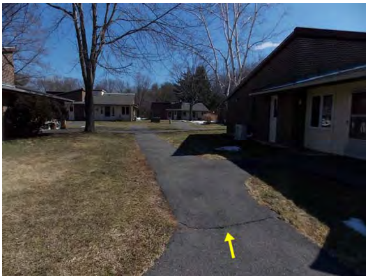
The secondary walkways are asphalt-paved. Note the cracked section.
