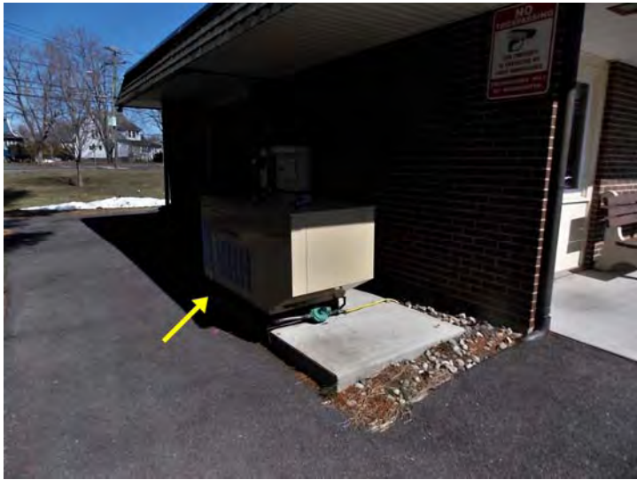
This propane-powered generator serves the community building.
